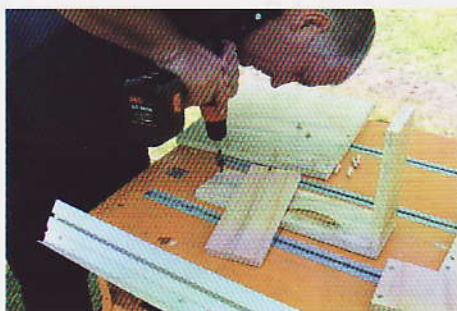
First assemble the sides to the backrest before attaching to the seat base.
